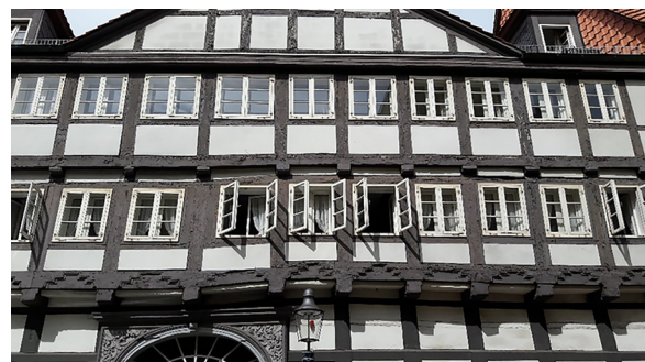
Fig. 1 Deformations due to creep effect in a wood structure (Braunschweig, Germany)
